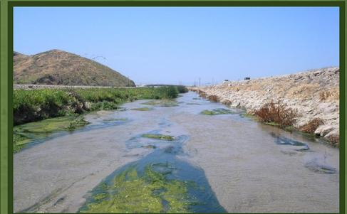
Figure 3. A soft-bottom channel with hardened sides. This stream in southern California is managed both for flood protection and to support groundwater infiltration.
