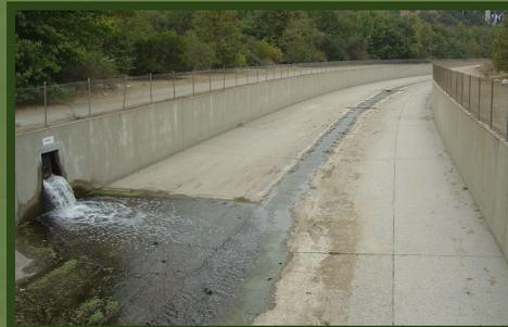
Figure 2. A concrete channel in Southern California, designed to move stormwater and protect surrounding property from flood damage.
