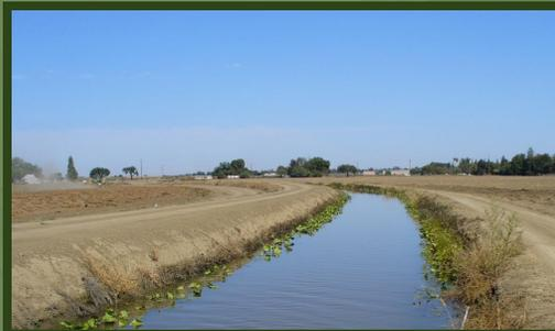
Figure 1. An earthen engineered channel in the Central Valley, primarily used to move water for agricultural supply.
