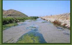
Figure 3. A soft-bottom channel with hardened sides. This stream in southern California is managed both for flood protection and to support groundwater infiltration.
